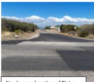
Newly paved section of Plateau Road, off Johnson Hill Main
